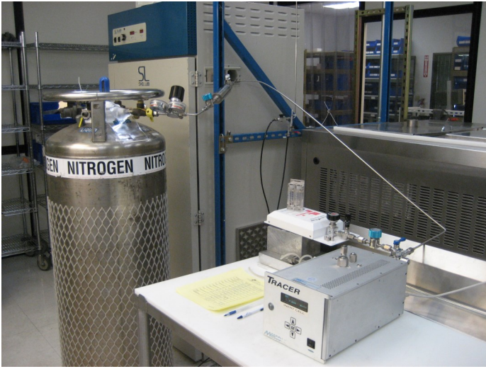
TEST SETUP: Purge gas and purifier, Meeco moisture analyzer connected to testing manifold, and test sample located in environmental chamber for elevated temperature test.
